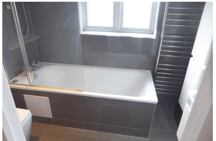
Panel enclosed bath with shower unit above, hand
